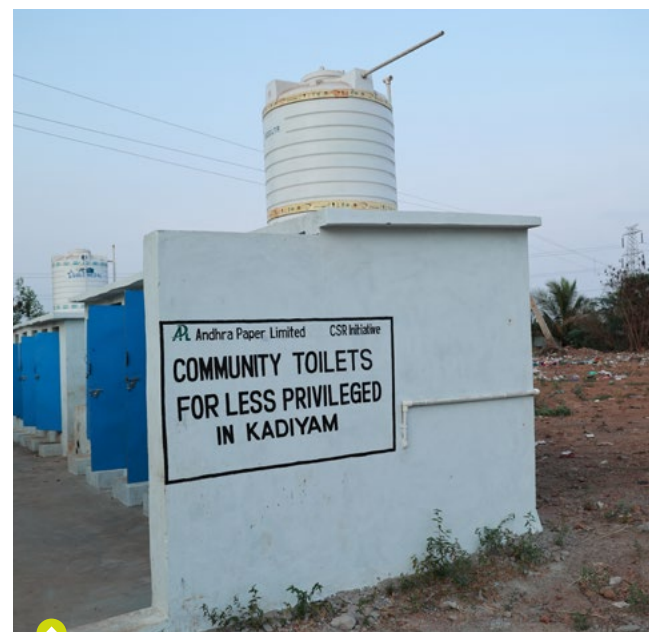
Constructed community toilets for under privileged in Kadiyam
