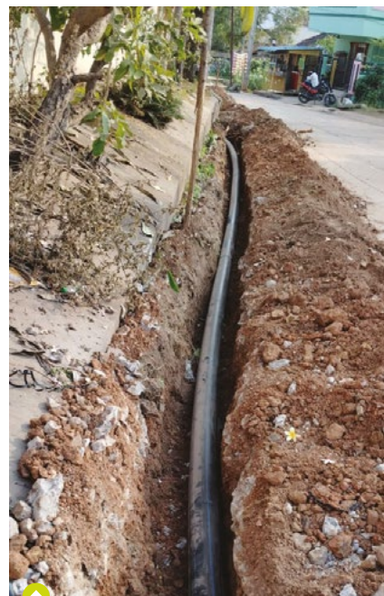
Laid pipelines in Kadiyam Village
